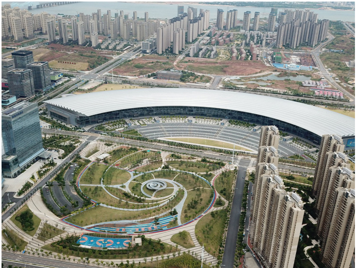
Nanchang Greenland International Expo Center
