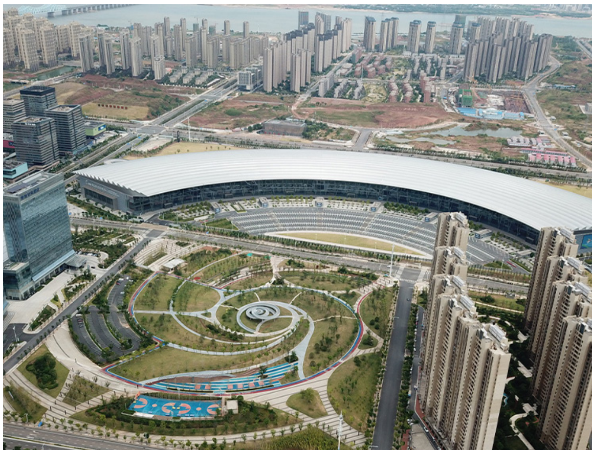
Nanchang Greenland International Expo Center
